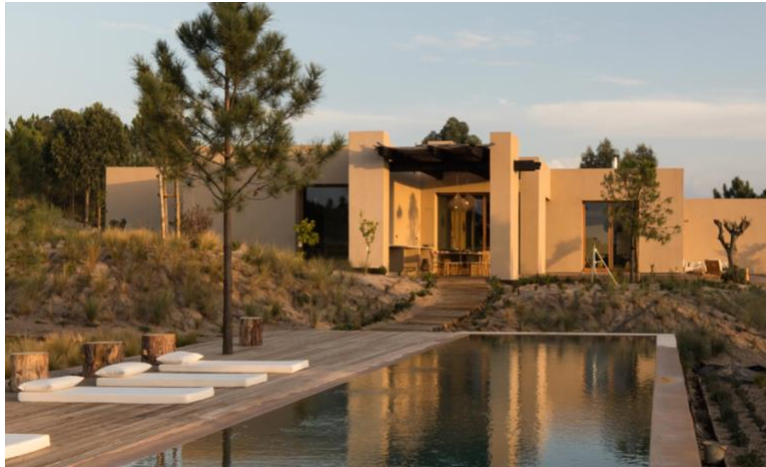
At Melides Art in Portugal, the private residences designed by Esteva i Esteva blend seamlessly with nature both in design and choice of material
